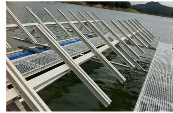
Fig. 5. Previous solar module support frame
