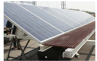
(b) Solar module support and foothold member
