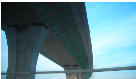
Fig. 1 PSC box girder bridge with RCFFT struts [2].
