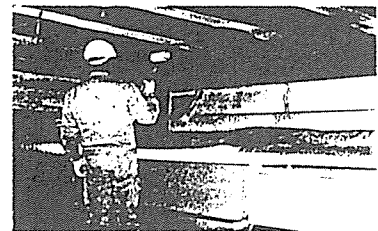
Fig. 6. Flexural Strengthening of Concrete Slab Using Carbon Fiber Tow Sheet[10]
