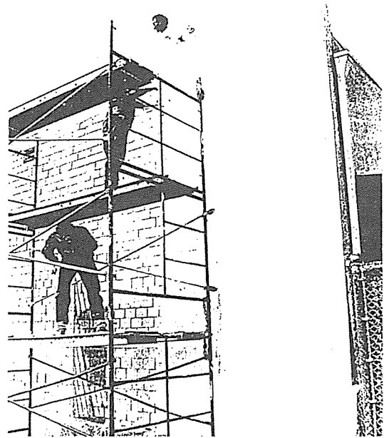
Fig. 10. Application of Composite Fabric for Wall Strengthening[28]
